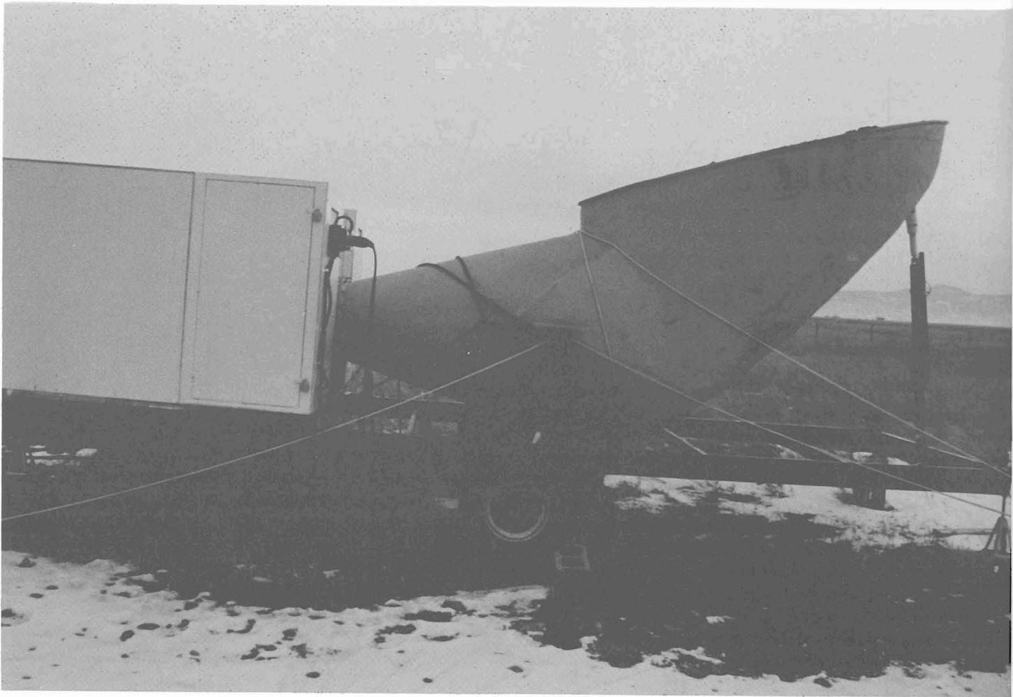
FIGURE 4. Prototype Main Transmitter Mounted on Movable Platform. The diameter of the exit portion of horn is approximately 2 meters.
